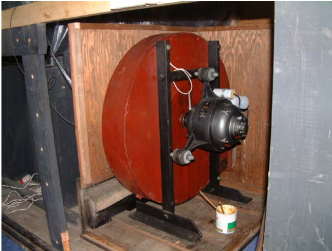
(above) The Blower and motor resided Jan 2006
