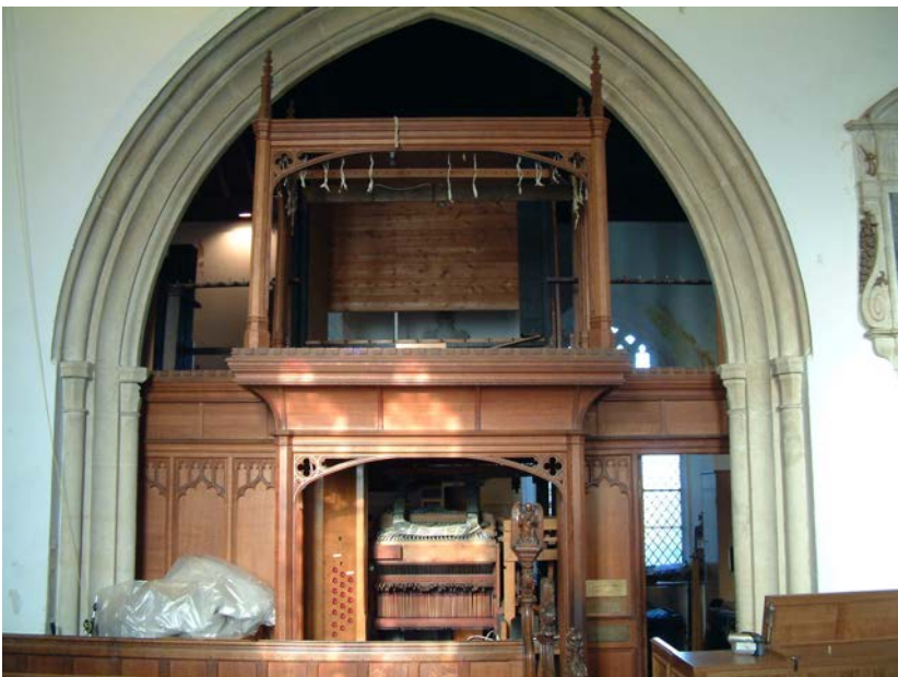
(Below) The cupboard was bare August 2005
